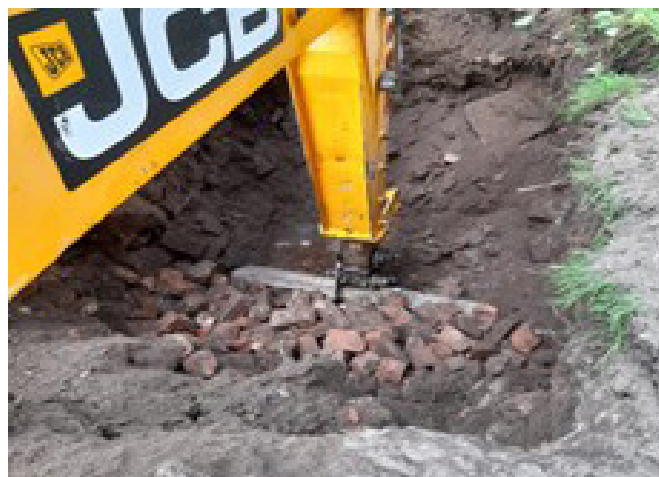
EXCAVATION OF DEEP HISTORIC PIT
