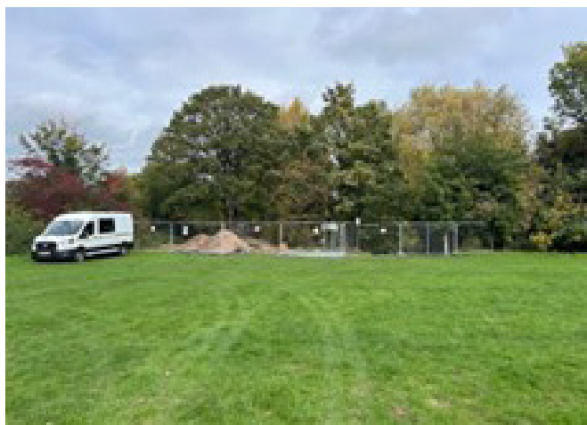
SITE SETUP INCLUDING FENCING AND CLEAR SIGNAGE
