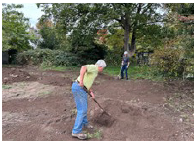
TOPSOIL SPREADING PRIOR TO GRASS SEEDING AT THE CONCLUSION OF THE PROJECT
