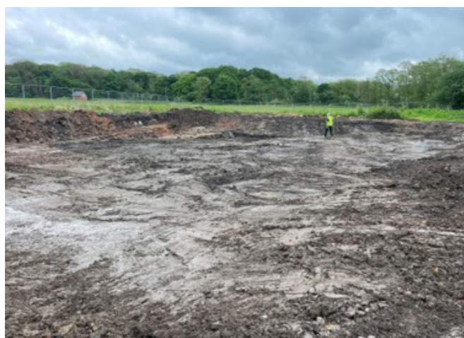
APC33 EXCAVATION EXTENT
