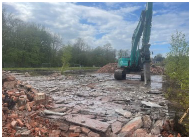
BREAKING OUT FLOOR SLAB AND UNDERGROUND STRUCTURES
