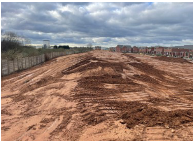
CLEAN COVER SYSTEM POS REINSTATEMEN
