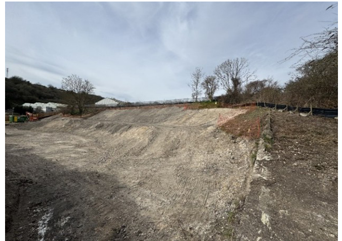
EXCAVATED WESTERN BATTER
