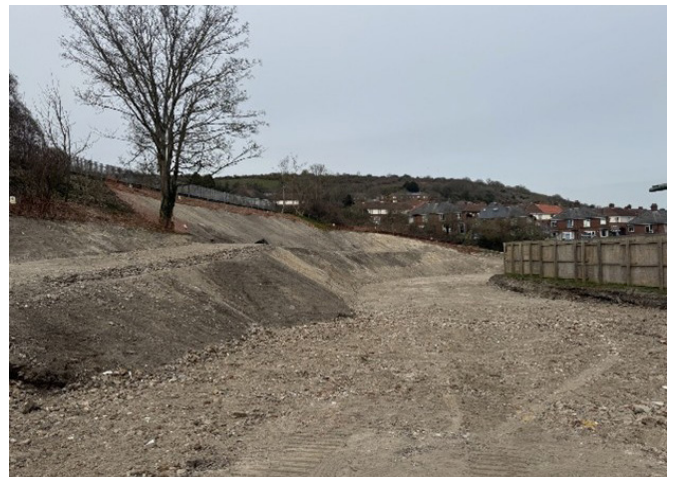
FINISHED FORMATION ACROSS SITE
