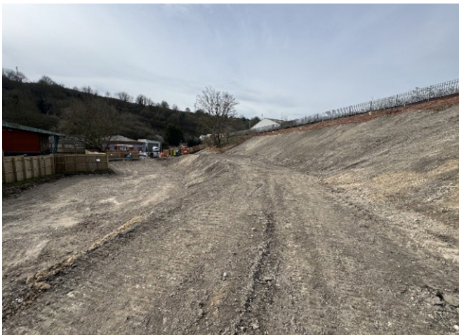
EXCAVATED WESTERN BATTER
