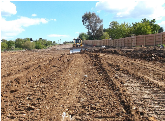
RE-PROFILING PRIOR TO SURCHARGING
