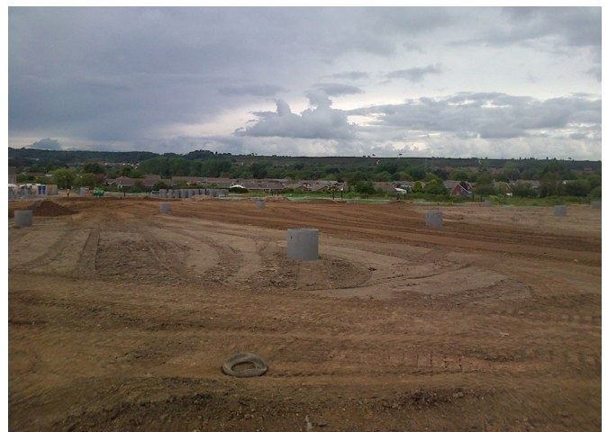
SITE RE-PROFILING IN COMPLETED PHASE
