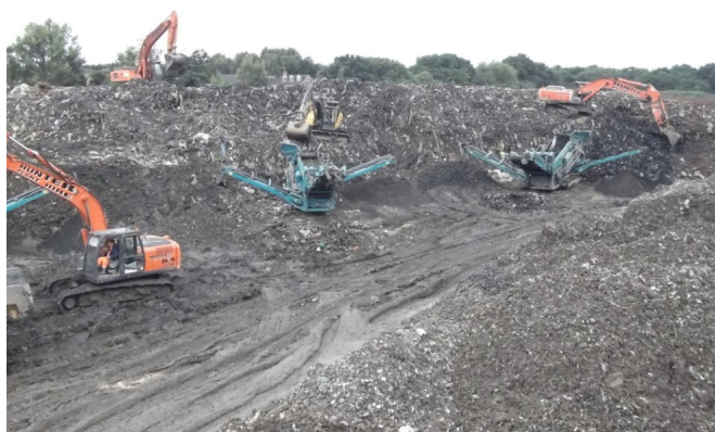
PROCESSING EXCAVATED LANDFILL WASTE USING PHYSICAL PROCESSING TECHNIQUES
