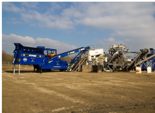
SOIL WASHING PLANT UTILISED FOR PROCESSING AND SEPARATING EXCAVATED LANDFILL WASTE
