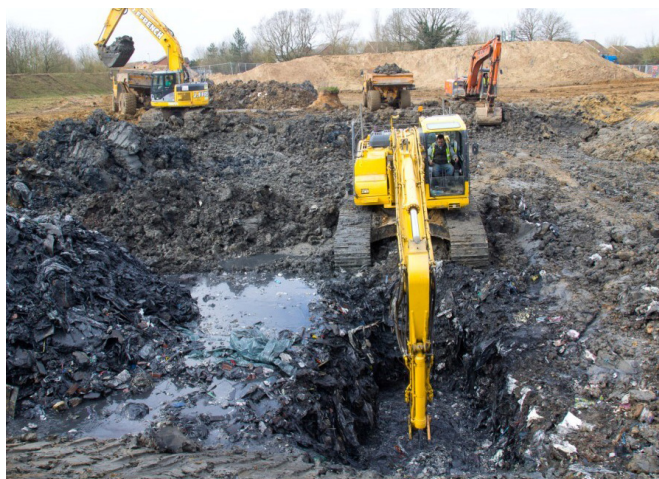
EXCAVATING WASTE FROM HISTORIC INDUSTRIAL/ COMMERCIAL LANDFILLS
