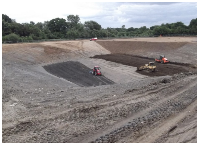
REINSTATEMENT OF MATERIALS WITHIN EXCAVATED VOIDS
