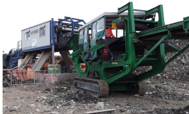
HANDPICKING LANDFILL WASTE TO SEGREGATE MATERIALS SUITABLE FOR REUSE ON SITE
