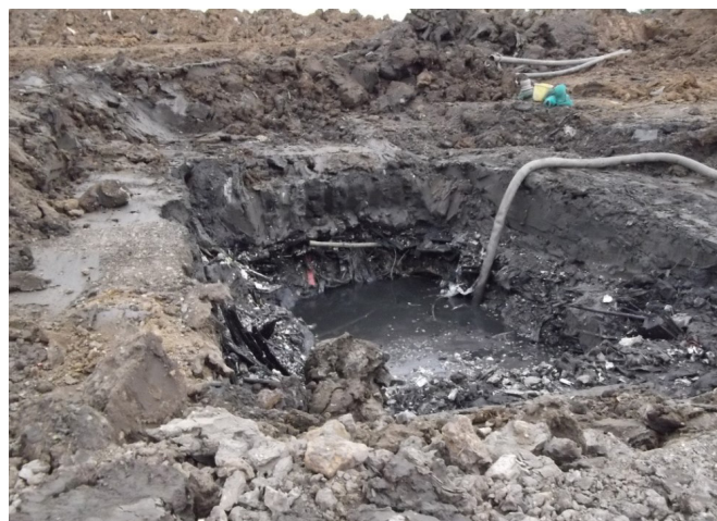
FORWARD DEWATERING FROM SUMPS
