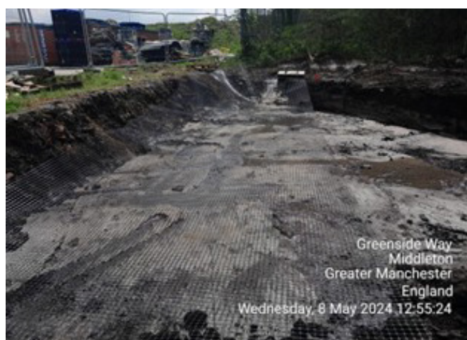
CONSTRUCTION OF SPINE ROAD WITH GEOTEXTILE
