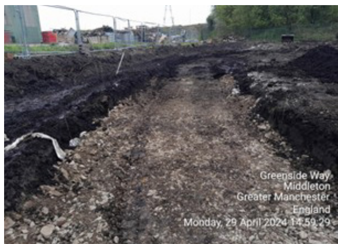
FINISHED CONSTRUCTION OF TRIAL PAD
