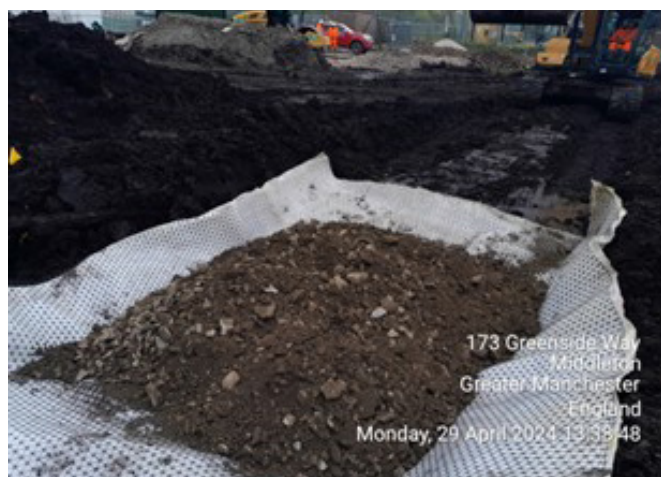
CONSTRUCTION OF TRIAL PAD
