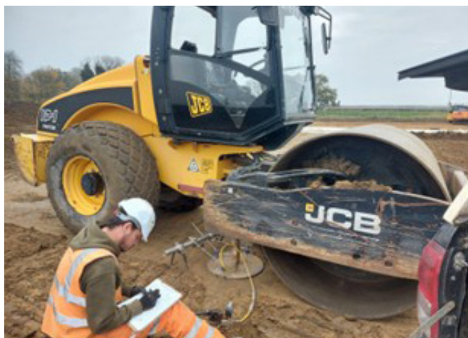
PLATE BEARING TESTING ON ROAD FORMATION
