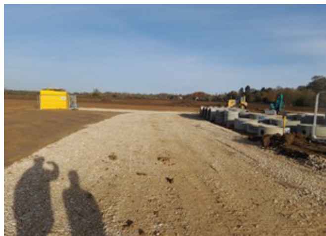
CAPPING STONE PLACED ON ROAD CORRIDOR
