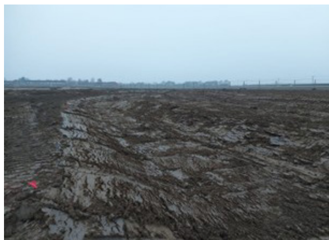
TOPSOILED TREATMENT POND
