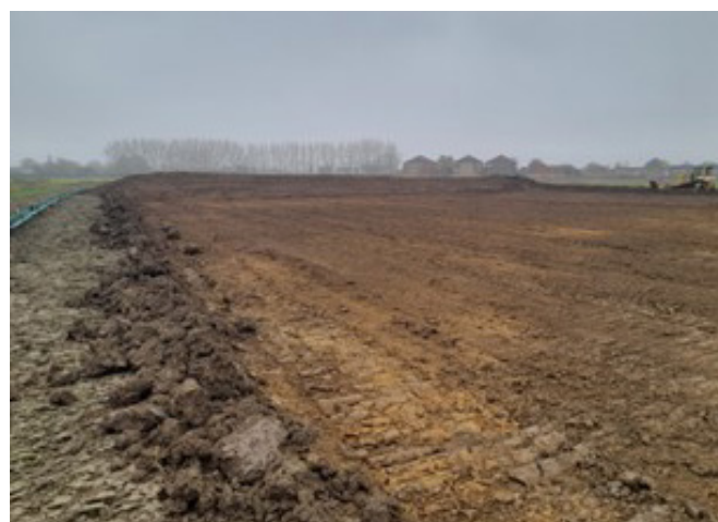
TOPSOIL STRIPPING
