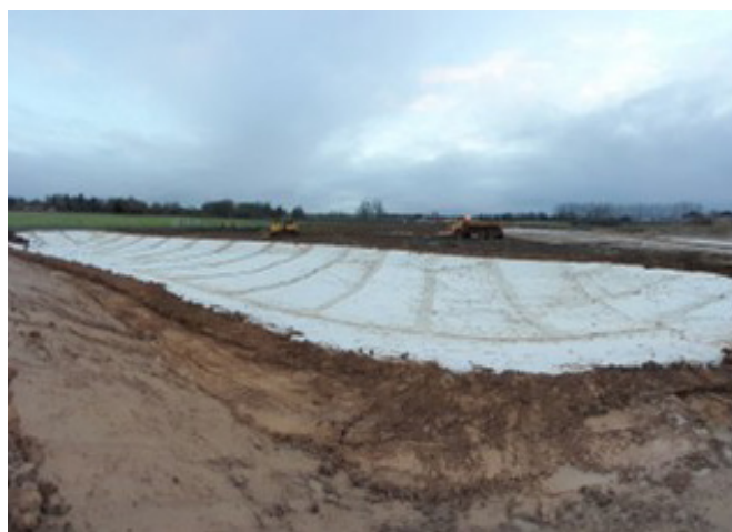
LINED TREATMENT POND
