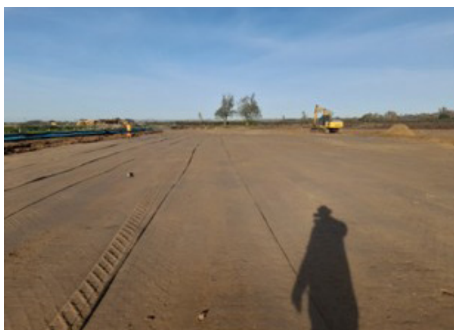
EARTHWORKS FILL TO DEVELOPMENT PLATFORM
