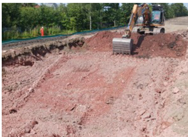
PLOT EXCAVATION, 1M BELOW FFL
