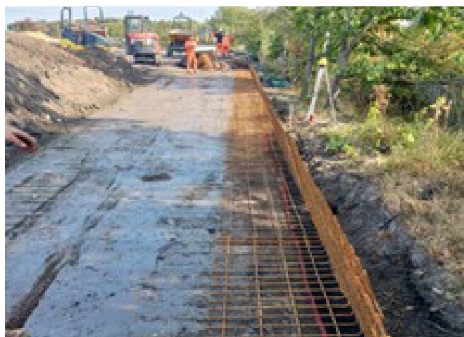
AB RETAINING WALL STEEL PANELS
