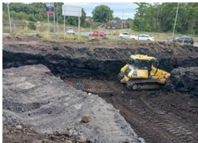
ROAD CORRIDOR ADDITIONAL EXCAVATION, SOFT SPOT BELOW 2M TURNOVER, ADDITIONAL 1M REQUIRED
