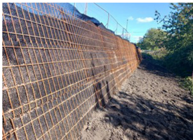
COMPLETED AB SLOPE RETAINING WALL FINISHED FACE
