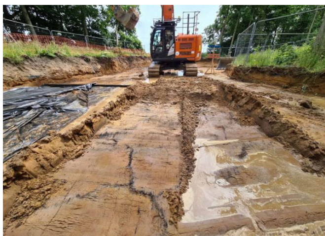
EXCAVATION OF SOFT SPOTS WHERE EARTHWORKS SUB-FORMATION UNSUITABLE FOR CONSTRUCTION
