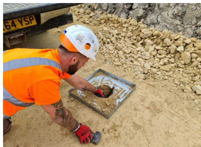
EARTHWORKS VALIDATED IN SITU BY SRD AND CBR TESTS
