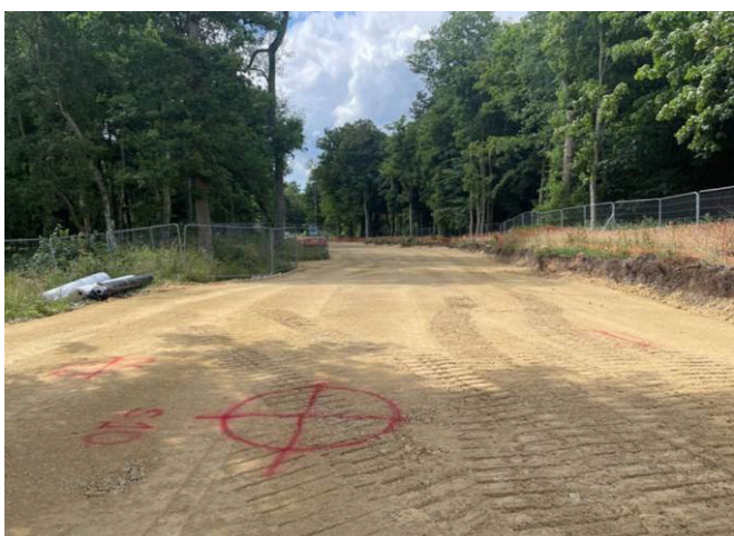
COMPLETED PRODUCT – TOP OF CAPPING LAYER
