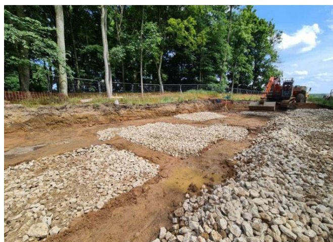
SOFT SPOTS EXCAVATED AND REPLACED WITH 6C IN ACCORDANCE WITH THE DESIGN
