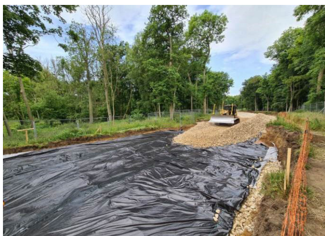
PLACEMENT OF GEOTEXTILE SEPARATOR LAYER OVER EARTHWORKS SUB-FORMATION LAYER FOLLOWED BY CLASS 6C MATERIALS
