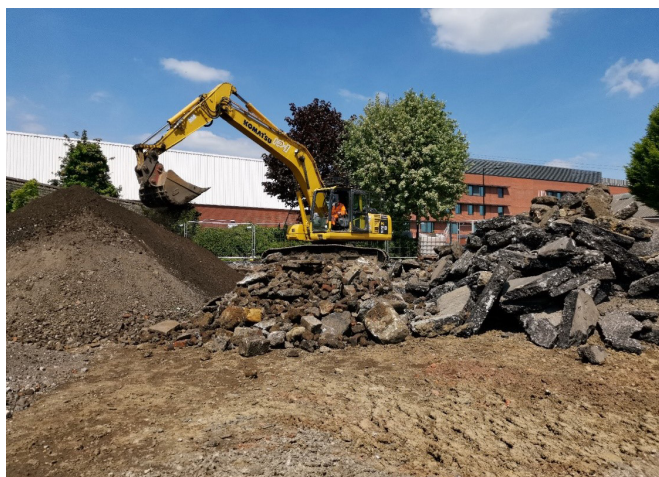
EXCAVATION AND PROCESSING OF SITE WON MATERIALS
