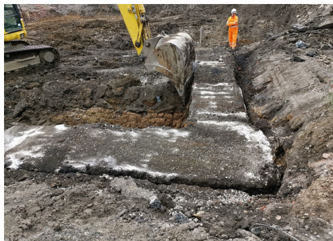
LARGE OBSTRUCTIONS UNSUITABLE FOR EXCAVATION WERE FIRST FULLY EXPOSED BY EXCAVATOR
