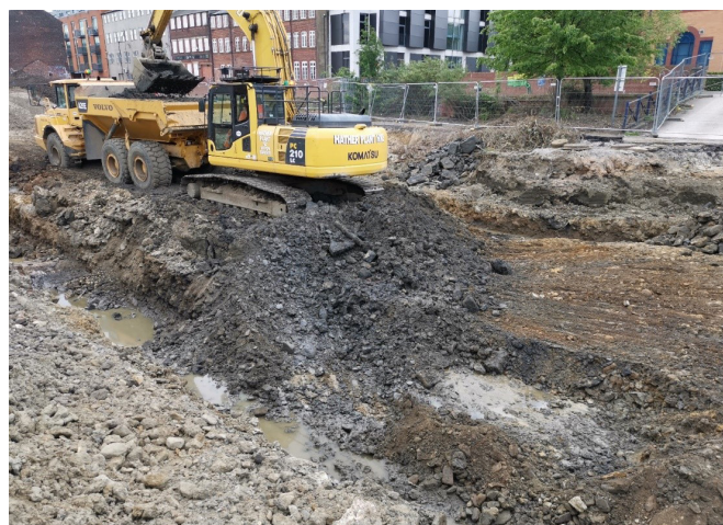
PRODUCT IMPACTED MADE GROUND WAS EXCAVATED FROM EXCAVATION CELLS TO STOCKPILE FOR OFFSITE DISPOSAL
