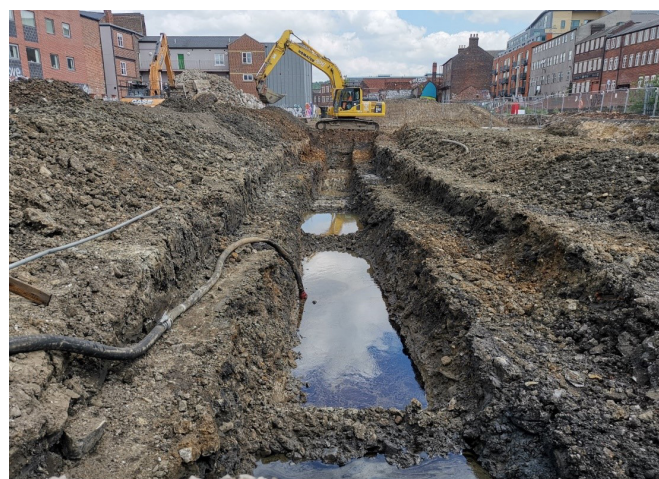
FORWARD DEWATERING TRENCHES WERE EXCAVATED TO RECOVER GROUNDWATER AND FREE PRODUCT IN THE LNAPL AREA.
