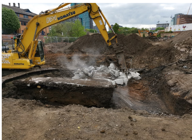
ONCE EXPOSED, LARGE OBSTRUCTIONS WERE BROKEN OUT BY EXCAVATOR USING MECHANICAL BREAKER. RUBBLE WAS LIFTED TO STOCKPILE FOR PROCESSING.
