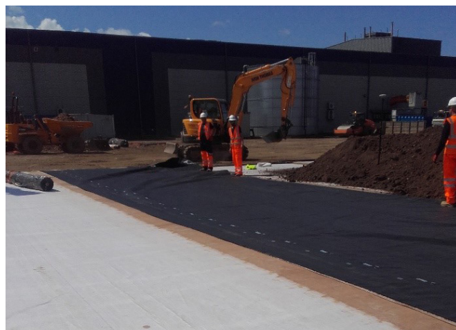
SEALING THE EDGES OF GCL
