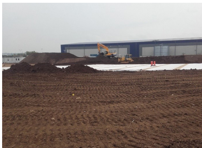
PLACEMENT OF TOPSOIL
