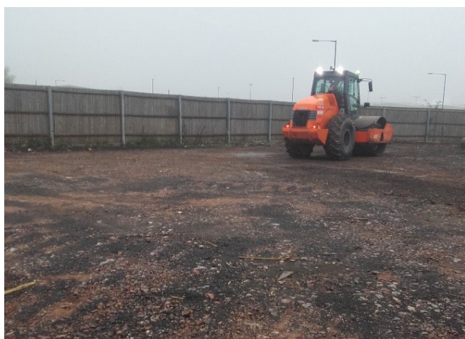
PREPARATION OF GROUND TO INSTALL GCL
