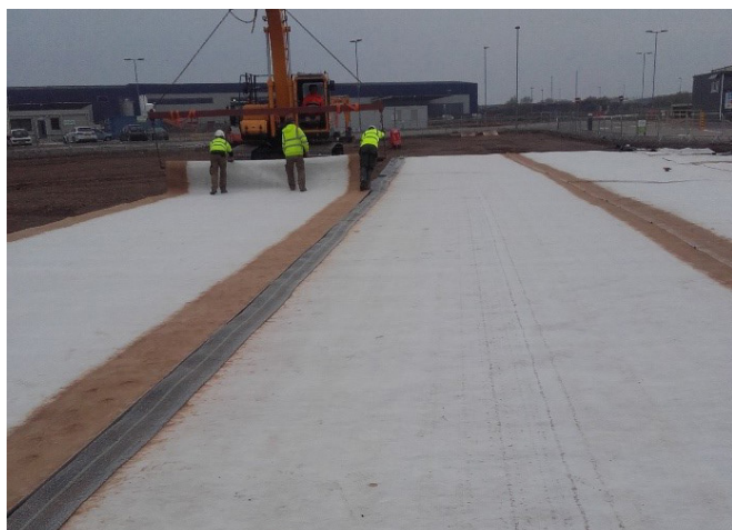
INSTALLATION OF GCL
