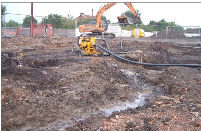
HYDROCARBON HOTSPOT REMOVAL PUMPING WATER AND FREE PHASE PRODUCT TO ON SITE WATER TREATMENT
