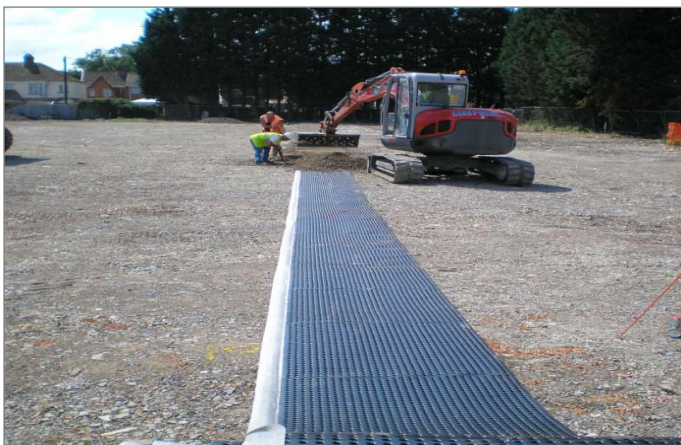
INSTALLING THE HORIZONTAL GEOCOMPOSITE COLLECTION SYSTEM BENEATH ASDA CAR PARK
