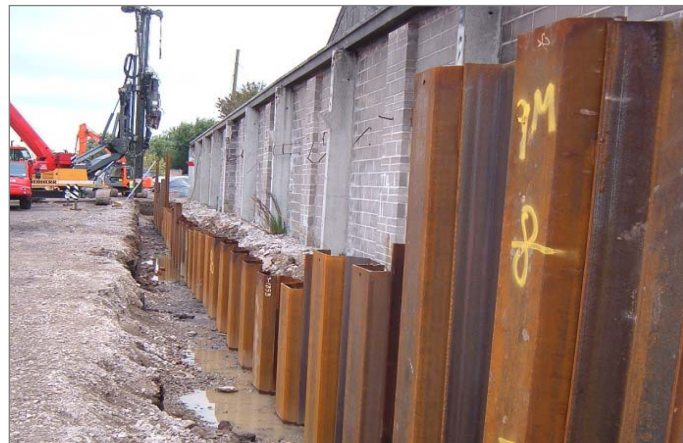
INSTALLING HYDRO BARRIER CUT OFF WALL TO PROTECT SITE FROM OFF SITE CONTAMINATION
