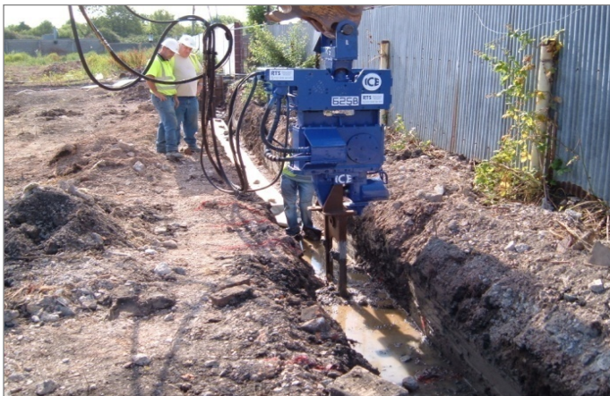
INSTALLING THE VERTICAL GAS CURTAIN AROUND THE INFILLED PITS TO PROTECT OFF SITE RECEPTORS
