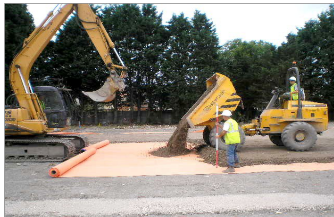
GASLAYING THE GEOTEXTILE MARKER LAYER OVER THE HORIZONTAL GAS COLLECTION SYSTEM
