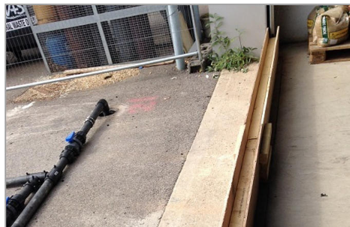
UNIT SECURED TO PREVENT UNAUTHORISED ENTRY
