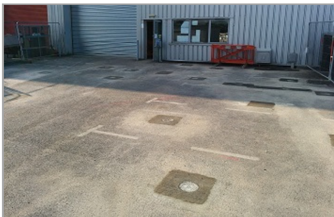
WELLS INSTALLED WITH COVERS
