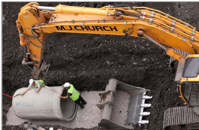
INSTALLATION OF DEEP DRAINAGE
