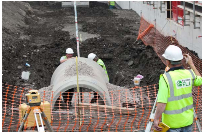
SETTING OUT OF DRAINAGE RUNS
