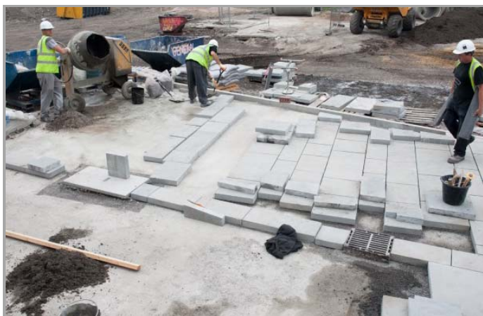
EXTERNAL FINISHING WORKS
