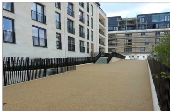
COMPLETED EXTERNAL WORKS
