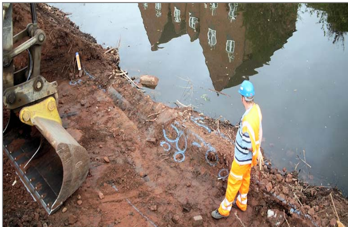
EXCAVATION OF JAPANESE KNOTWEED
