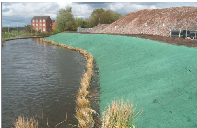
COMPLETED CANAL BANK WITH BIOMAT, HYDROSEEDED AND COIR ROLL
