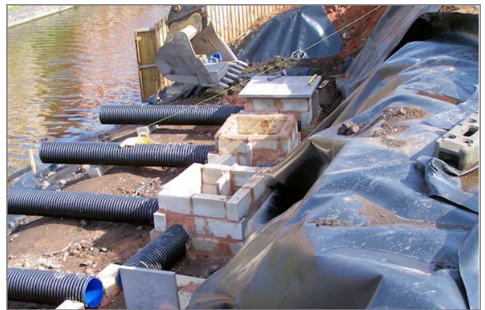
CONSTRUCTION OF NEW ARTIFICIAL BADGER SETT
