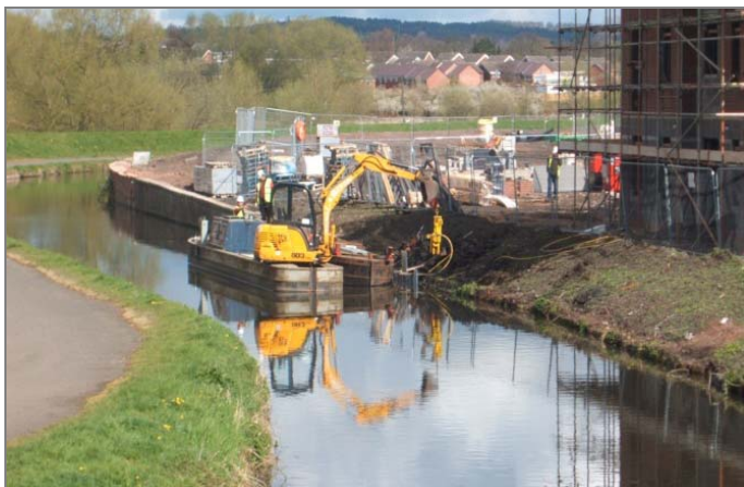
BARGE ON CANAL UNDERTAKING WORKS
