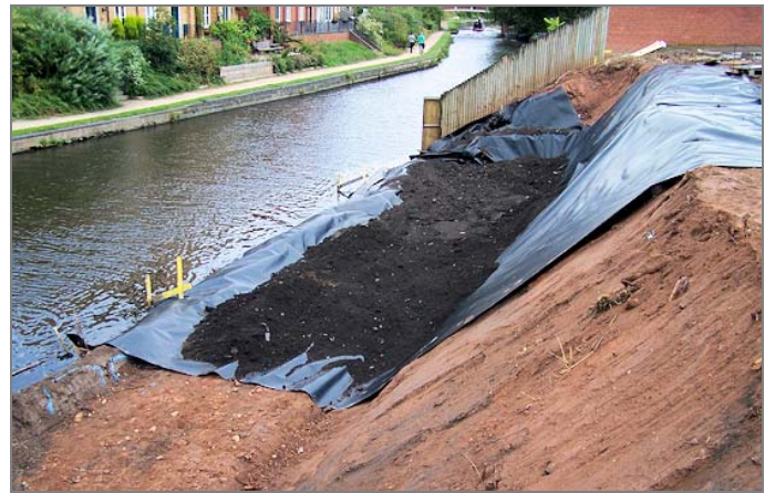
REINSTATEMENT OF CANAL BANK WITH ROOT BARRIER
