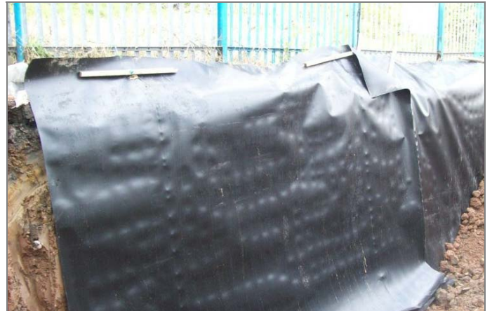
HDPE BARRIER WAS DROPPED INTO EXCAVATION USING PULL CORDS
