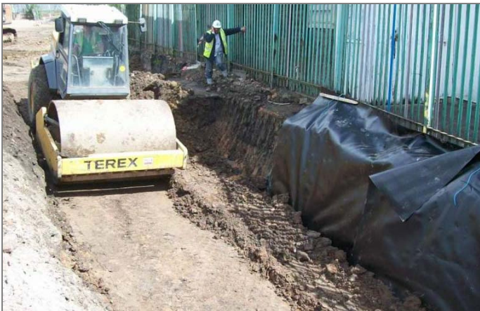
EXCAVATION REINSTATED WITH CLEAN SITE WON MATERIALS AND COMPACTED IN 300MM LAYERS
