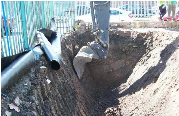
EXCAVATION DOWN TO 3.5MBGL FOR KNOTWEED BARRIER
