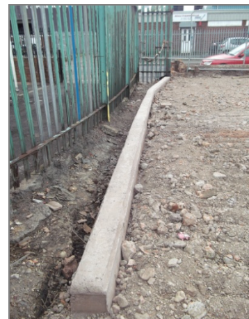
CONCRETE BEAM WHICH SECURES THE TOP EDGE OF THE MDPE KNOTWEED BARRIER
