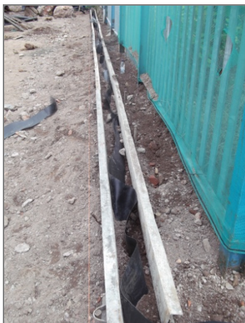
FORMWORK PLACED TO TOP OF KNOTWEED BARRIER READY FOR CONCRETE
