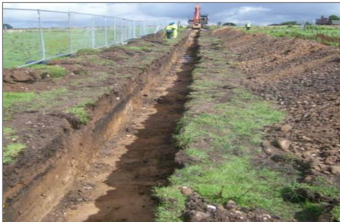
EXCAVATED LEADER TRENCH
