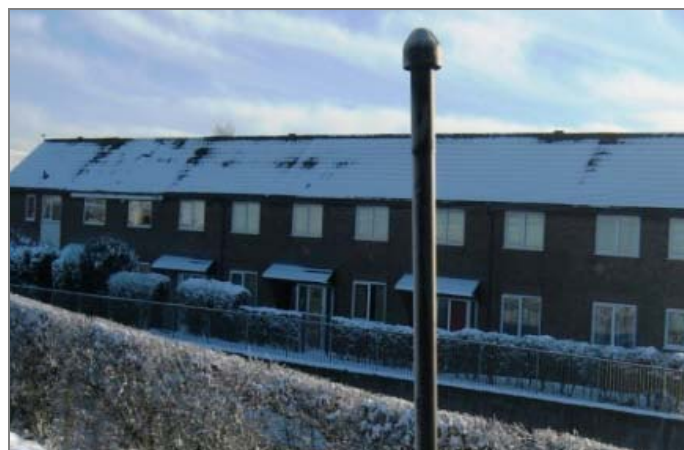
COMPLETED VENT BOLLARD
