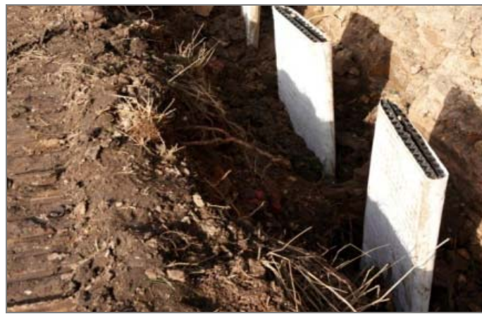
INSTALLED SECTION OF NODES
