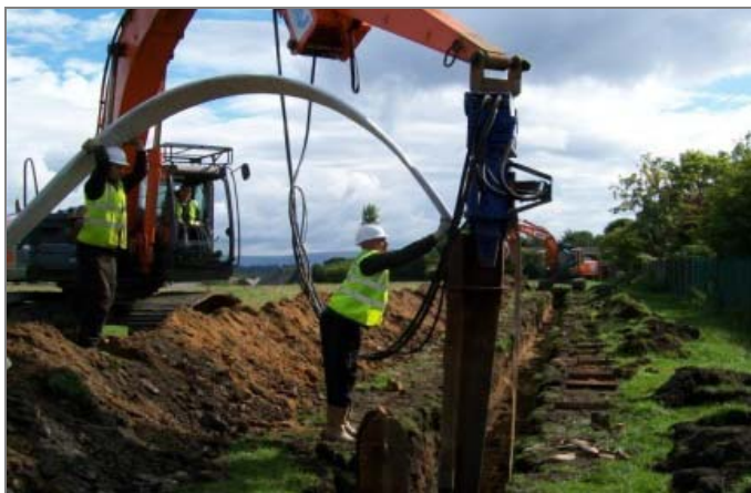
INSTALLATION OF GEO-COMPOSITE NODES
