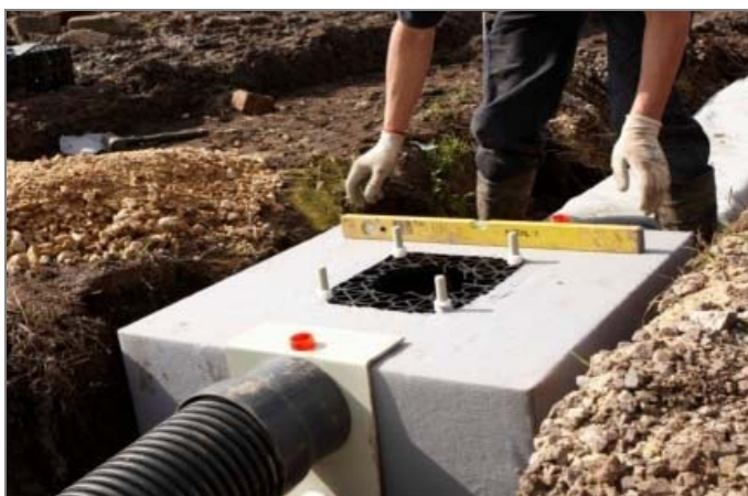
VENT STACK BASE
