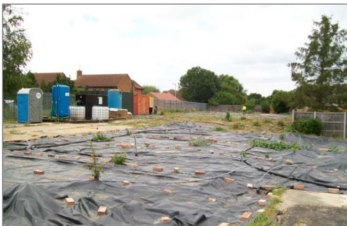
INSTALLATION OF VAPOUR EXTRACTION LINES WITH HDPE COVER
