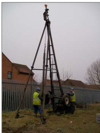
INSTALLATION OF EXTRACTION WELLS
