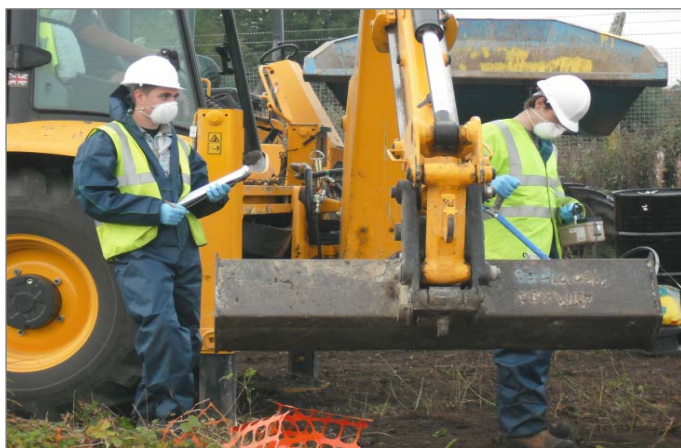
SCANNING EXCAVATED MATERIAL FOR SENTENCING
