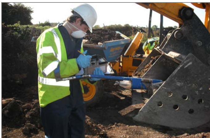
SCANNING EXCAVATED MATERIAL FOR SENTENCING
