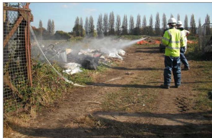
DAMPING DOWN PRIOR TO EXCAVATION
