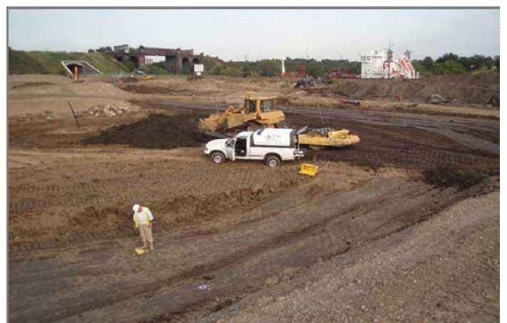
VERIFICATION UTILISING NUCLEAR DENSITY GUAGE
