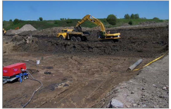
EXCAVATED TO REDUCED LEVEL AND PREPARING FOR IN-SITU SYSTEM INSTALLATION
