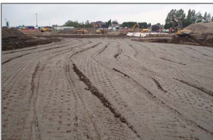
RE-ENGINEERED CLAYS FOLLOWING COMPACTION BY BACKFILLING, COMPACTION AND GEOTECHNICAL
