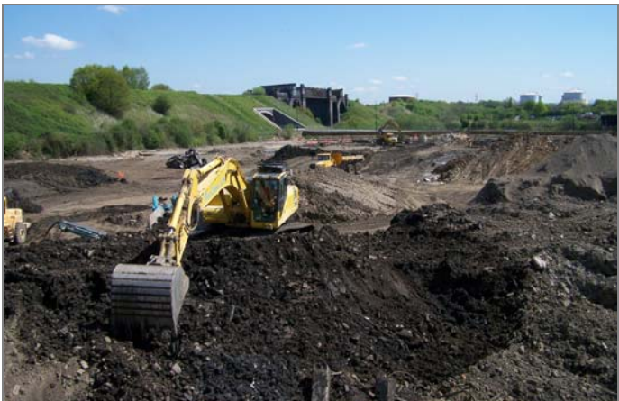
EXCAVATING FROM STOCKPILE FOR SCREENING AND BIOPREPARATION
