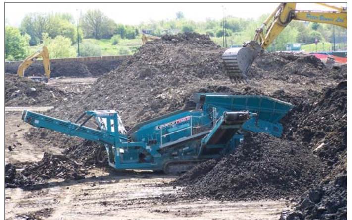
SCREENING MATERIAL PRIOR TO VERIFICATION AND BACKFILL
