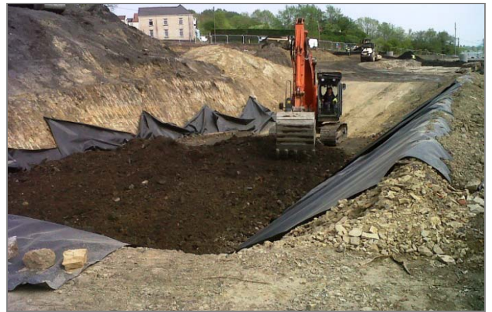
LEVELLING OUT SOILS IN CELL
