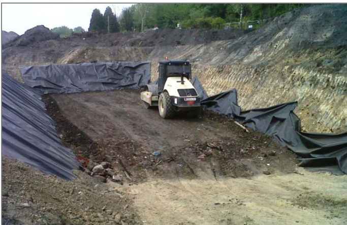
COMPACTION OF SOILS WITHIN CELL
