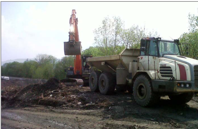
LOADING KNOTWEED INFESTED SOILS
