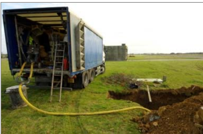
FOAM FILLING BURIED PIPE
