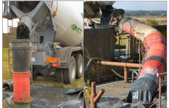
FILLING TANK WITH GROUT
