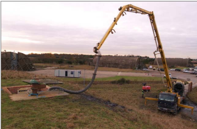
FILLING TANK WITH GROUT USING TELESCOPIC BOOM PUMP
