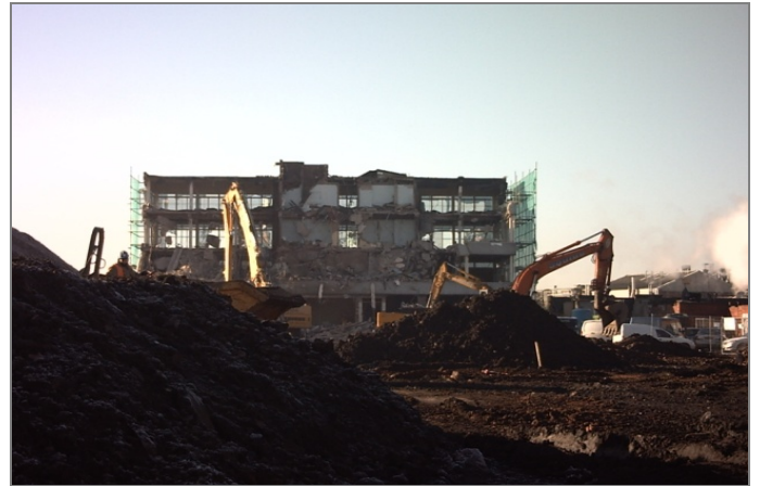
DEMOLITION OF OFFICE BLOCK USING LONG REACH EXCAVATORS WITH HYDRAULIC SHEARS
