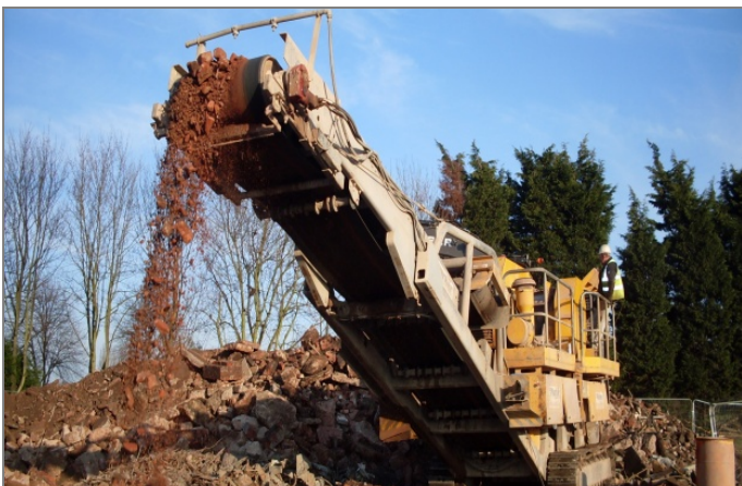
CRUSHING AND PROCESSING DEMOLITION MATERIAL TO SECONDARY 6F2 AGGREGATE
