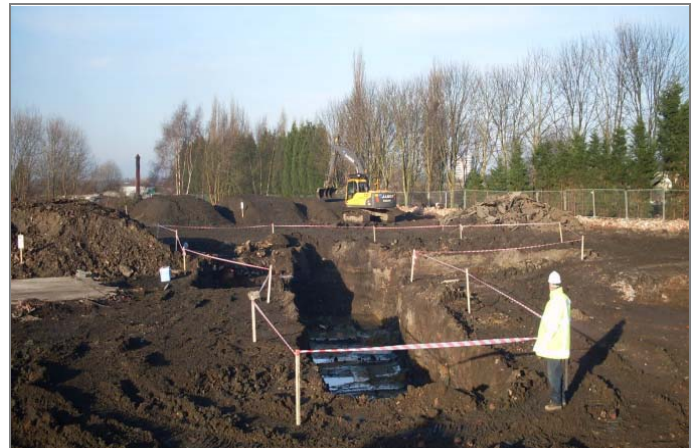
EXCAVATION OF HOTSPOT MATERIAL AND CONSTRUCTION OF TREATMENT BEDS
