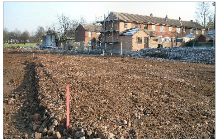
REINSTATEMENT OF SITE-WON MATERIAL TO FINISH LEVELS AND PILING MATS
