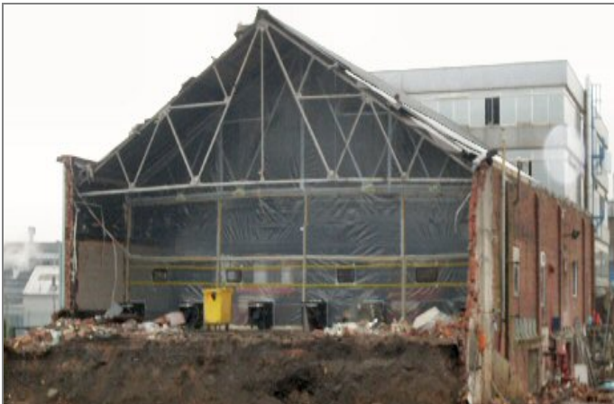
CONTROLLED REMOVAL OF NOTIFIABLE ASBESTOS FROM BUILDINGS PRIOR TO DEMOLITION
