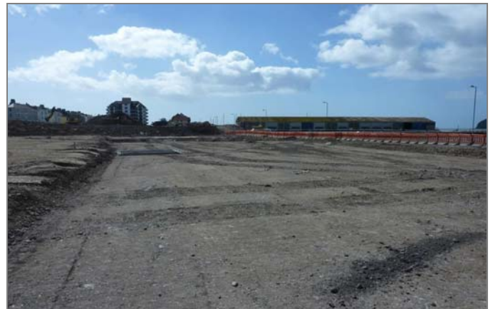
COMPLETED STABILISED SECTION WITH CAPPING LAYER
