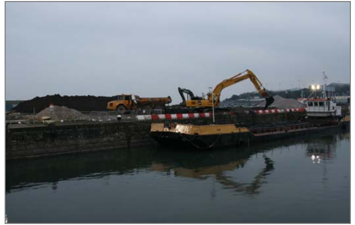
UNLOADING OF DREDGINGS TO QUAYSIDE (24HR OPERATION)
