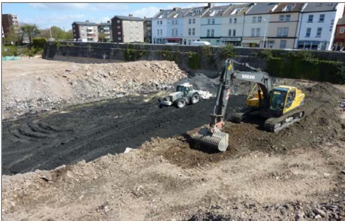
STABILISATION OF DREDGED MATERIAL
