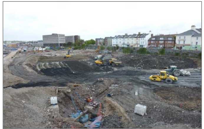
EXCAVATION OF LAGOONS
