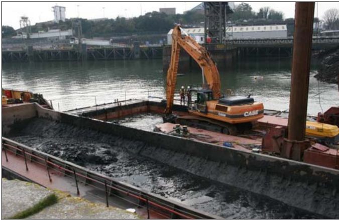
EXCAVATION OF DREDGINGS FROM HARBOUR
