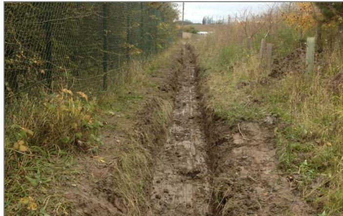
NEW TRENCH FOR TOE DRAINAGE INSTALLATION
