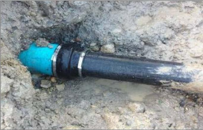
REPAIR TO FORMER LANDFILL CAP DRAINAGE
