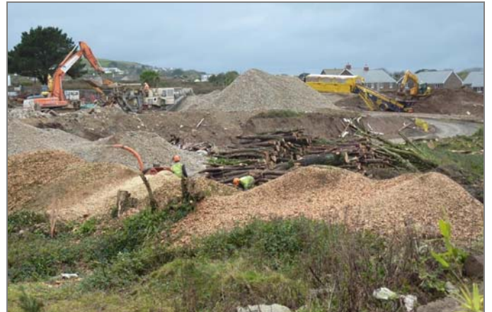
SITE CLEARANCE WORKS INCLUDING TREE FELLING
