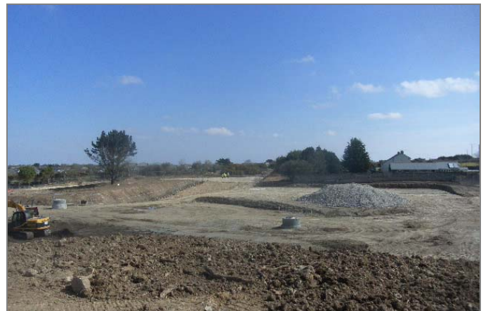
COMPLETED SITE PROFILED FOR DEVELOPMENT
