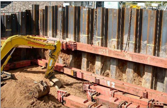
INSTALLATION OF SUPER TANK BRACING
