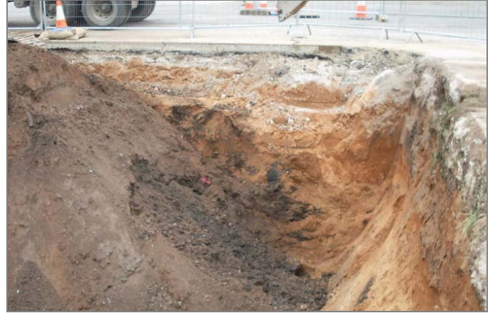
DISPOSAL OF CONTAMINATED SOILS
