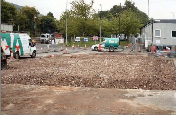
PREPARATION OF PILING MAT
