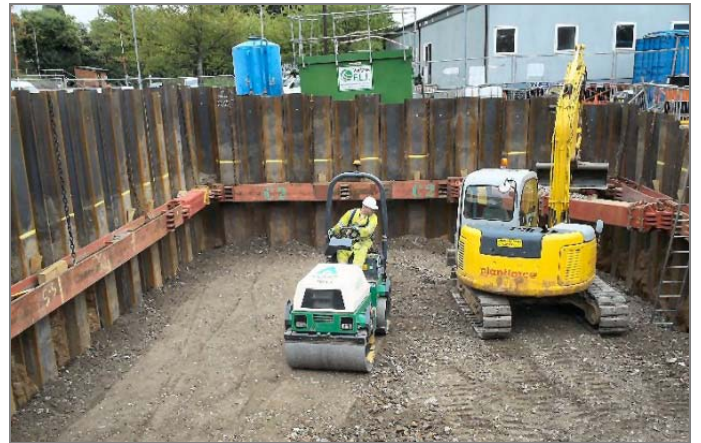
BACKFILL WITH IMPORTED STONE
