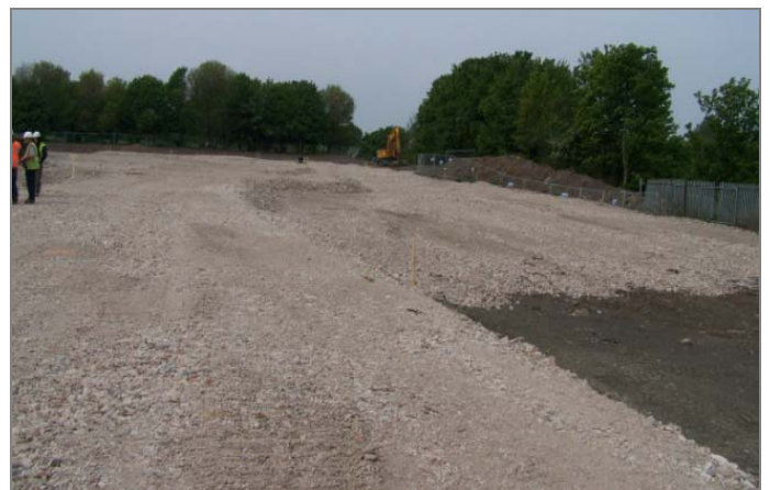
REINSTATEMENT OF SITE WON MATERIAL TO FINISH LEVELS
