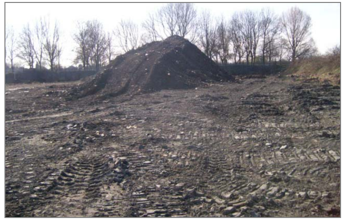
CONSTRUCTION OF BIOREMEDIATION
