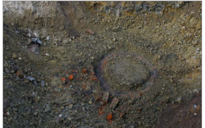
MINE WORKING INVESTIGATIONS INCLUDED LOCATION OF HISTORIC MINESHAFT KNOWN TO BE ON SITE
