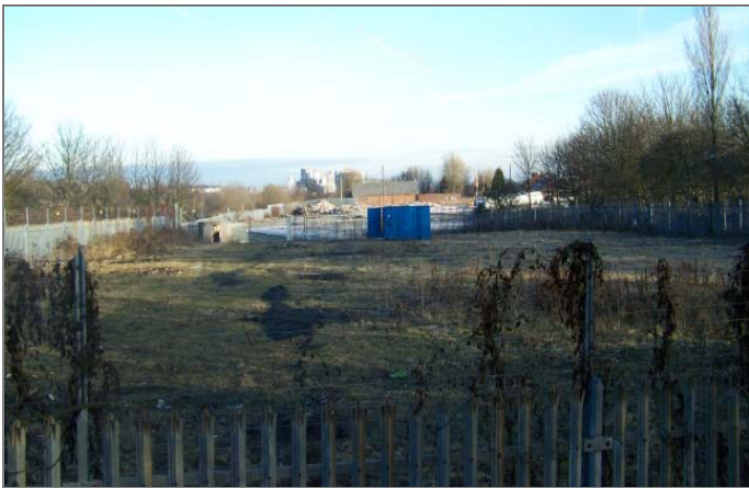
BEFORE WORKS COMMENCED
