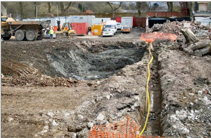
EXCAVATION OF CONTAMINATION FROM AROUND TANKS WITH LIVE MARKED CABLE
