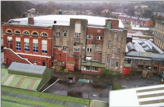
THE MILLS PRE DEMOLITION
